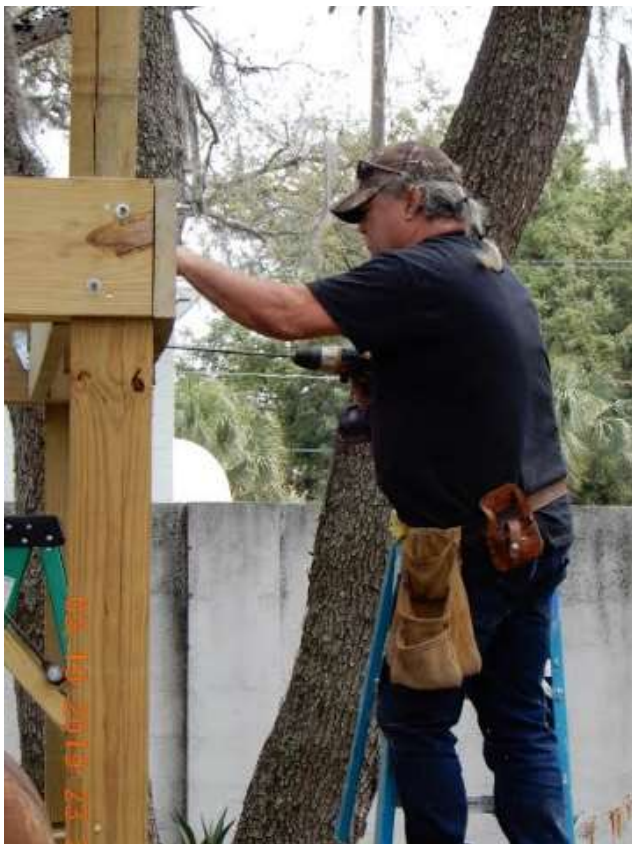
W.: Dennis Gomes working on the Grilling structure
